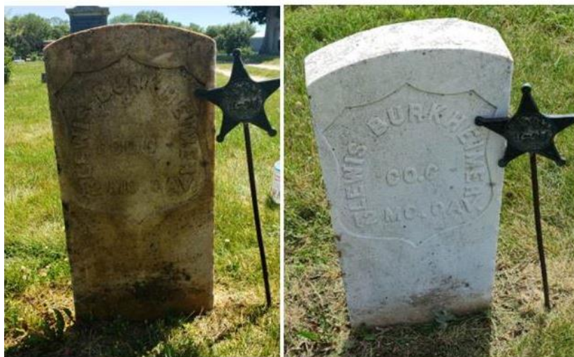
We were pleased to see that the chemical known as D2 worked as well on gravestones as we had heard. This one changed from grimy to glistening in under one week and with very little effort.
